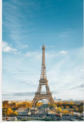
Eiffel Tower Wrought-iron lattice tower on the Champ
